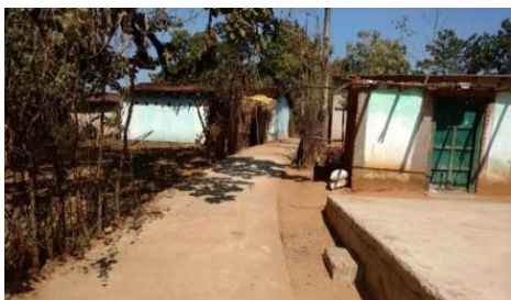
Road constructed in Ichak gram panchayat
